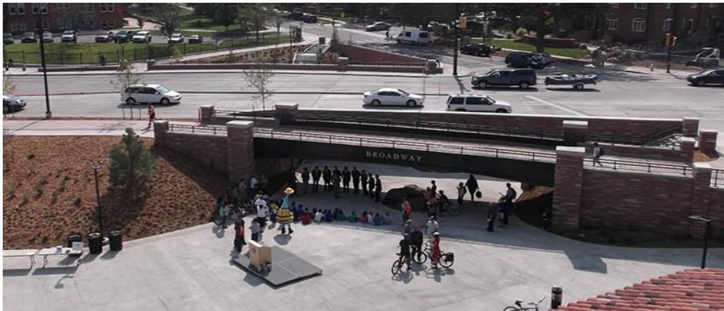
Figure 2 Broadway underpass, CU Boulder
